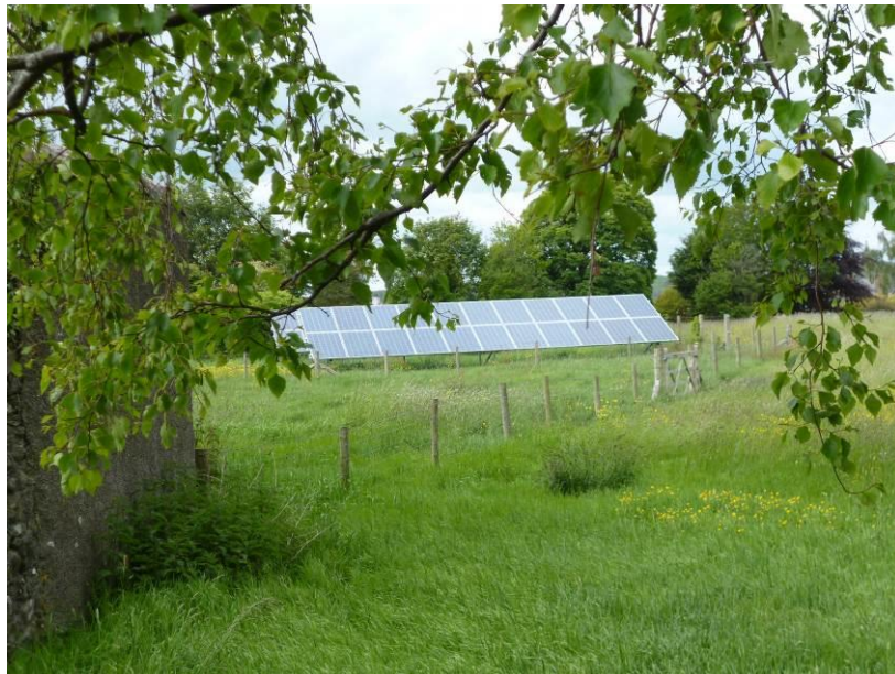
Fig.8: photovoltaic array in adjoining field
